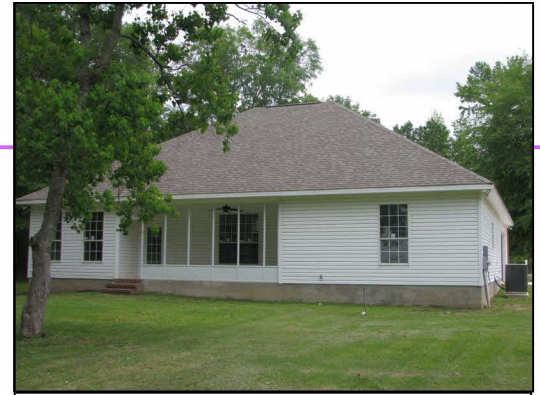
Back view of main home. Screened porch area.
