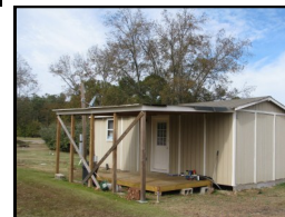
Workshop with bathroom, it's own septic system and power.
